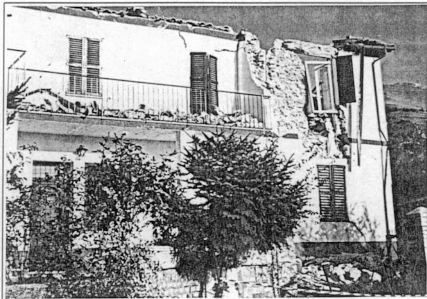
Figure 3: Collapse of the two-story building rubble masonry, in the settlement of Cesi.
